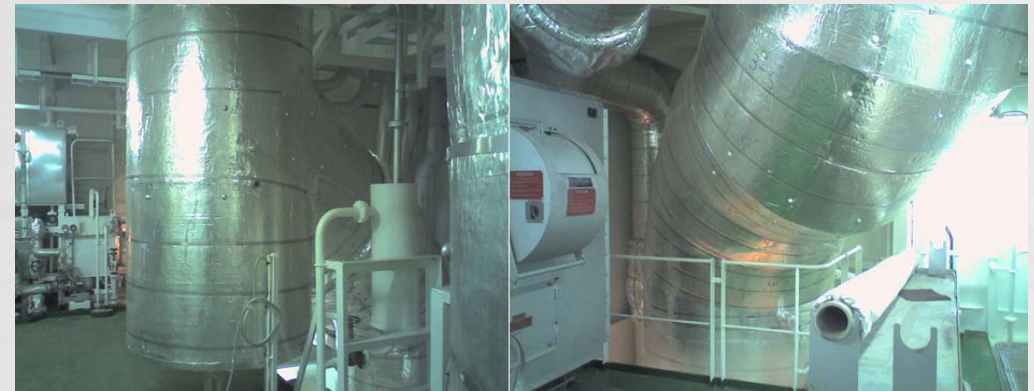
▶ Exhaust Gas Pipe, Elbow Cover (72")
